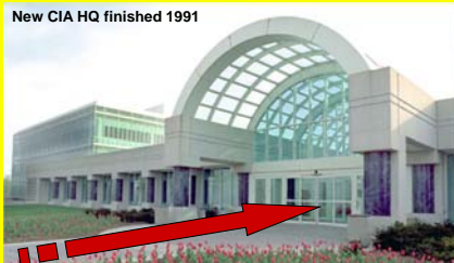
New CIA HQ finished 1991
